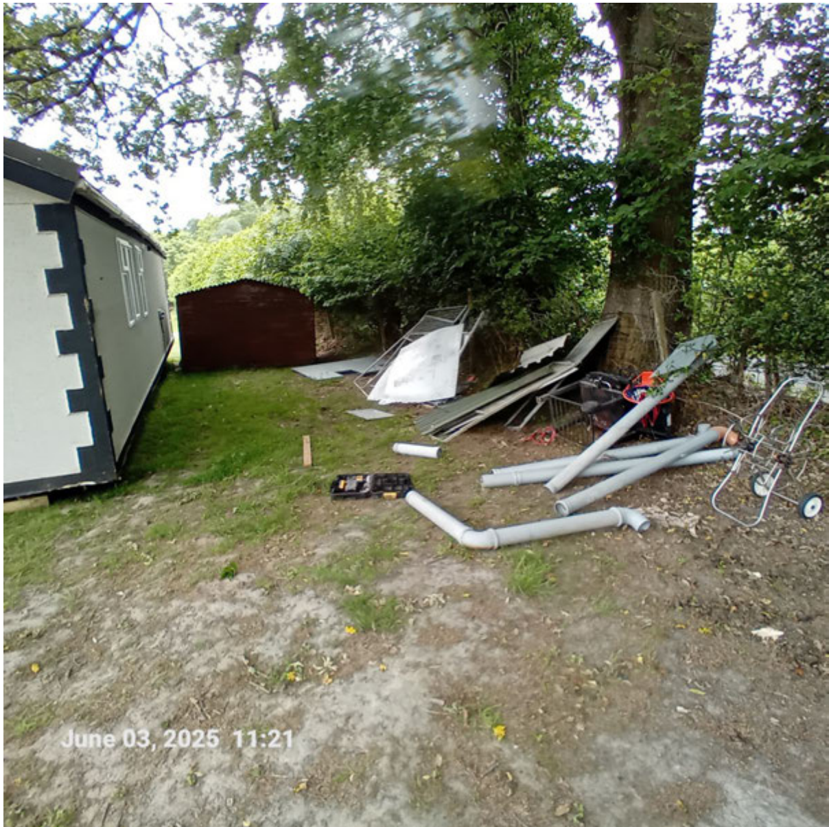
AC/72 Materials behind the 2 nd Mobile home and shed south of the other mobile home.
