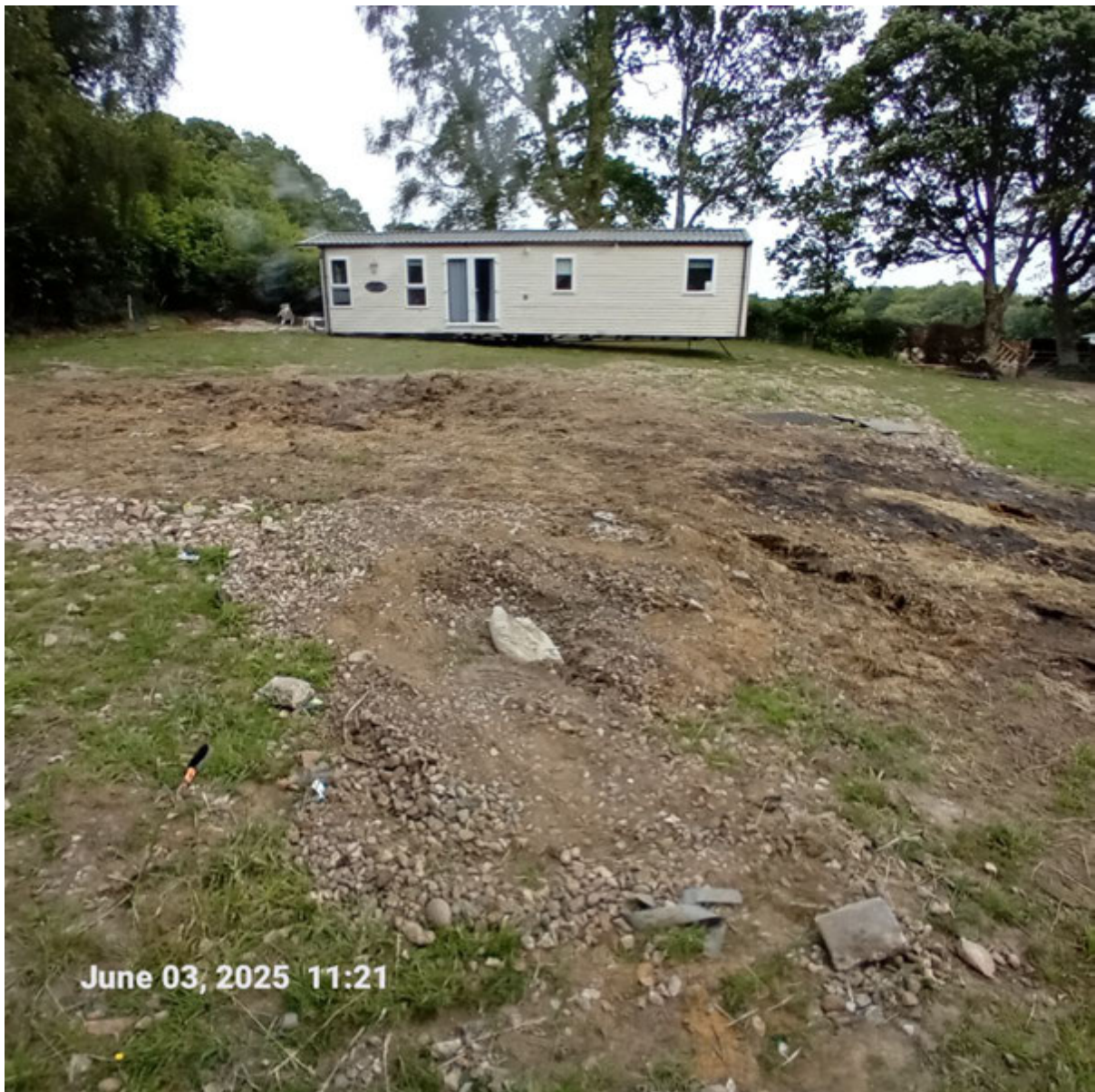
AC/67 Mobile home in northeast corner and hardcore on ground
