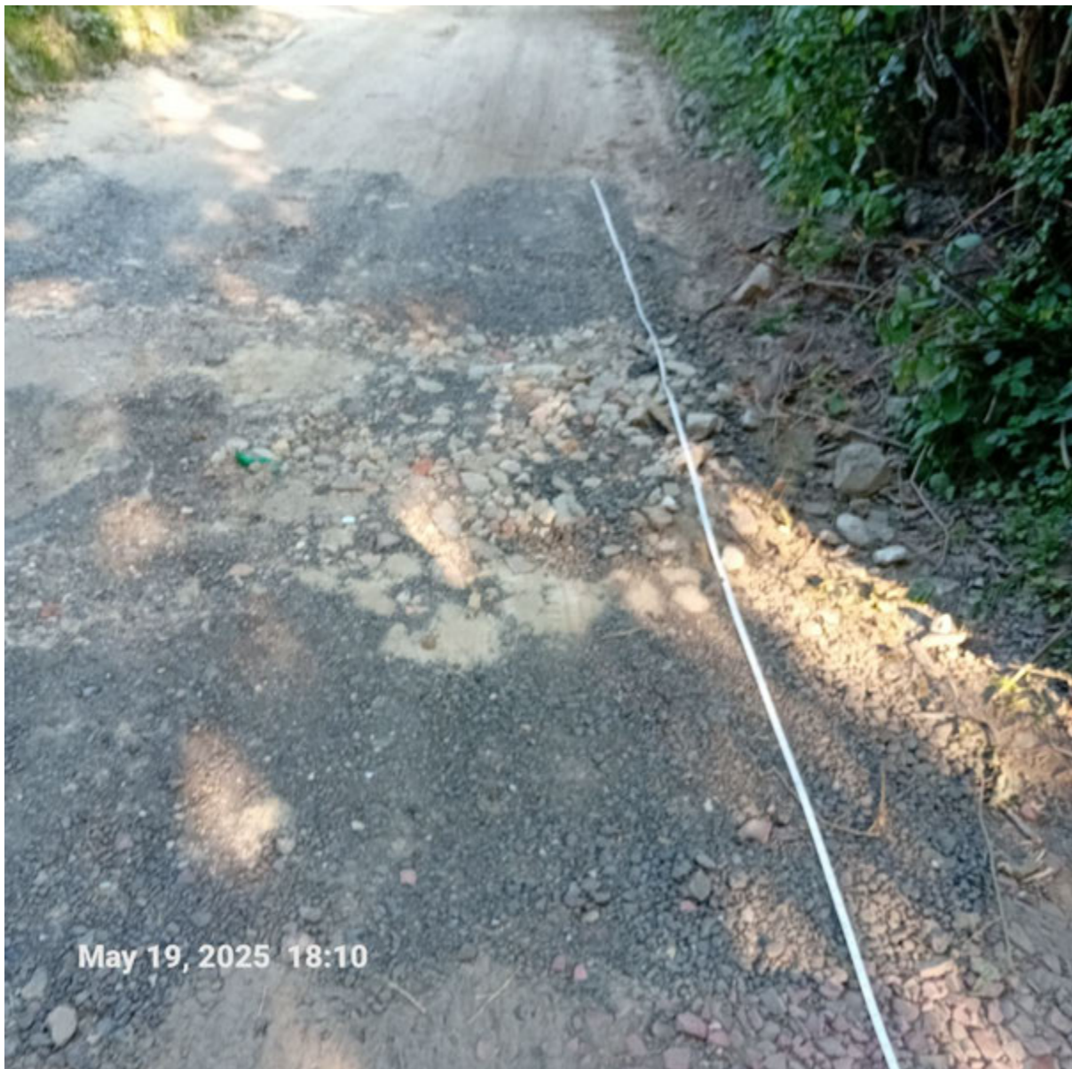
Exhibit AC/23 New hardcore laid for the track into the land
